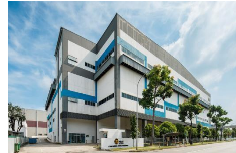
8 Tuas Avenue 20, Singapore
