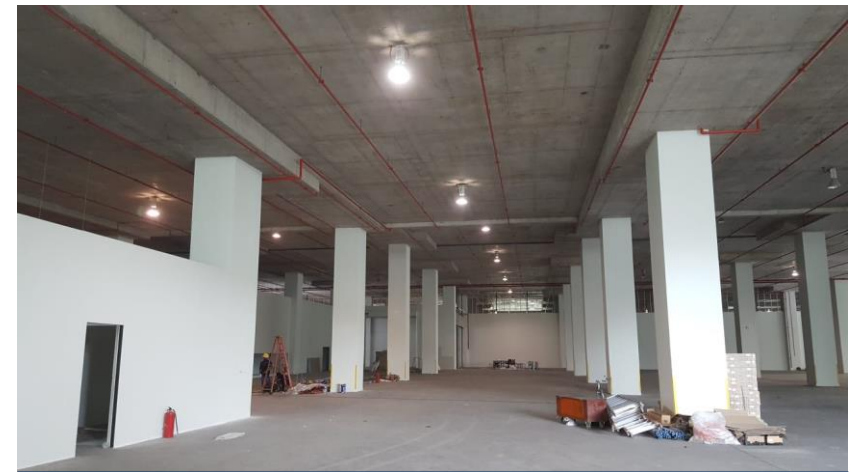
AEI Works in progress at ALOG Gul LogisCentre
