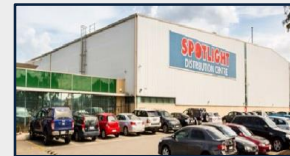
19 217 – 225 Boundary Road, Laverton North
