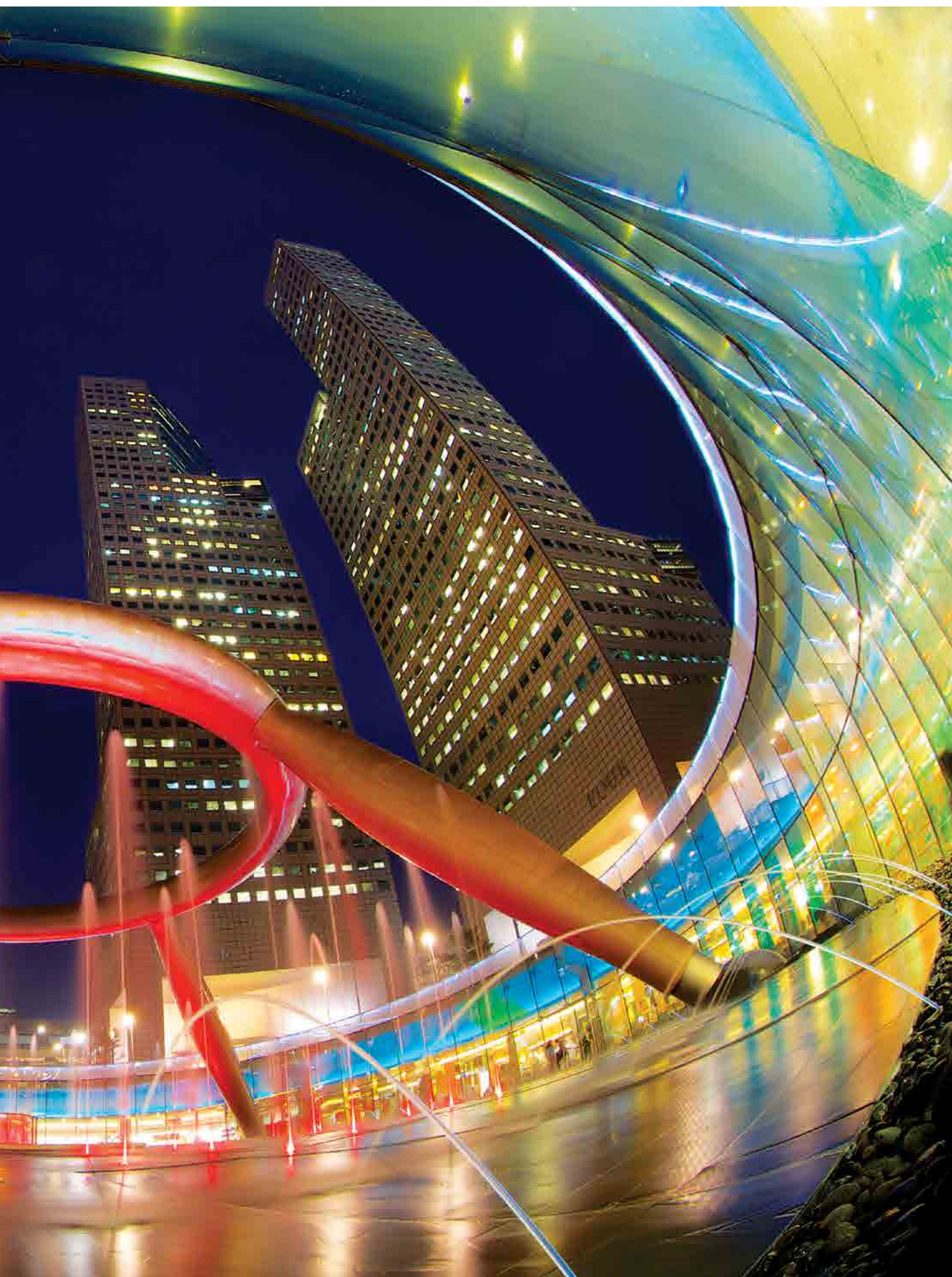
Suntec City Office and Suntec City Mall, Singapore
