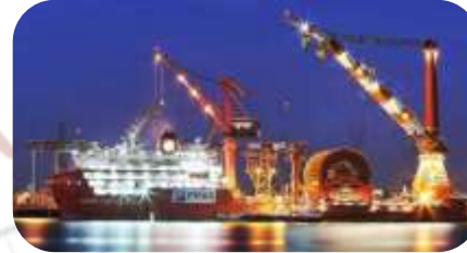
Installation of Multi-layer System ("MLS")
