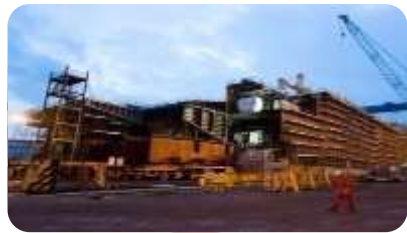
Superstructure of vessel completed
