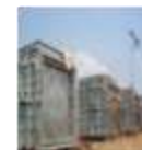
Industrial Fabrication (Diverters for refineries and power plants)
