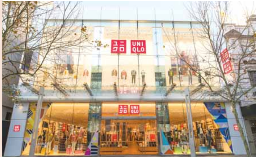
The completed asset redevelopment of Plaza Arcade presented a revamped façade facing Murray Street Mall and houses anchor tenant UNIQLO.
