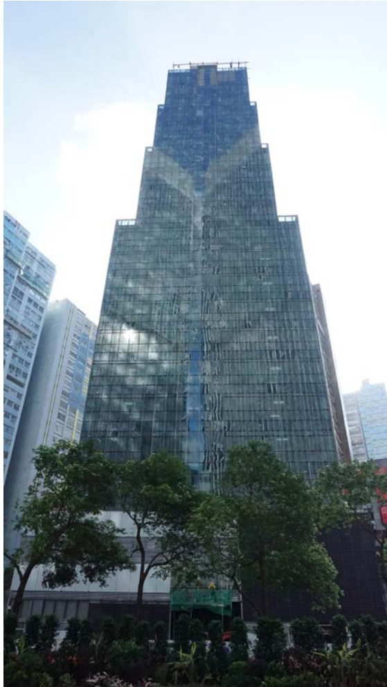
Existing site undergoing construction
