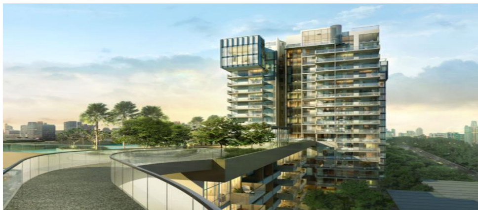
Sennett Residence, Singapore
