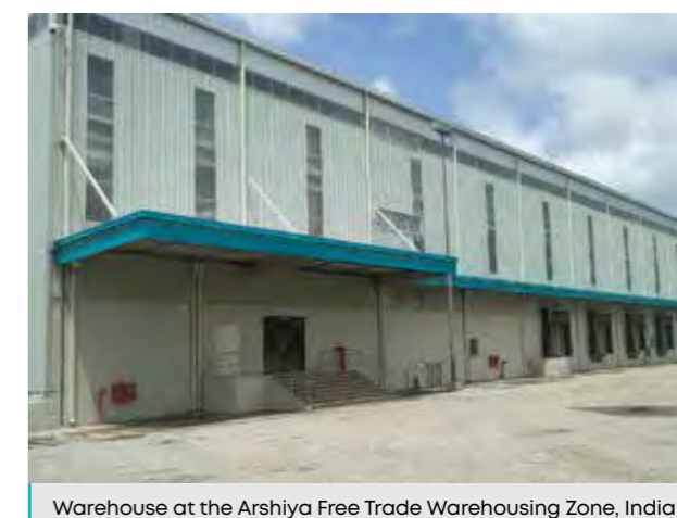
Warehouse at the Arshiya Free Trade Warehousing Zone, India
