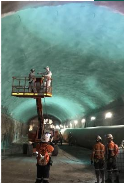
Waterproof membrane being applied in NorthConnex tunnel
