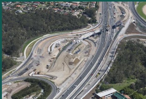
Gateway Upgrade North construction continues
