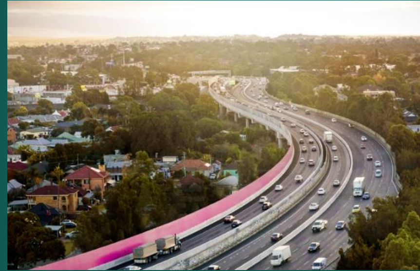
Completed M4 widening – Stage 1A of WestConnex
