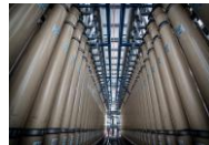
Keppel Seghers Ulu Pandan NEWater Plant
