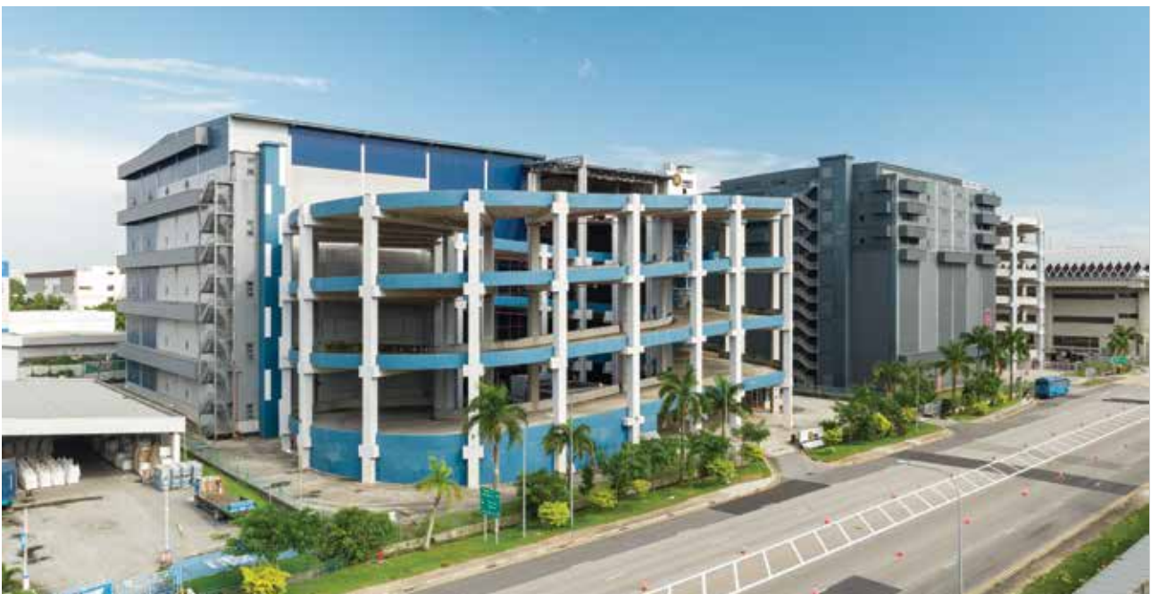
30 Tuas West Road, Singapore
