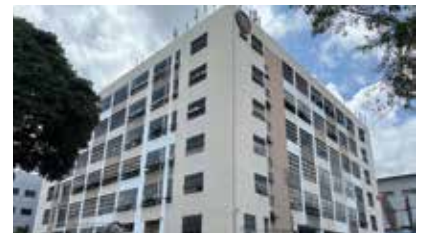
19 61 Yishun Industrial Park A
