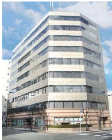
Utsubo East Building
