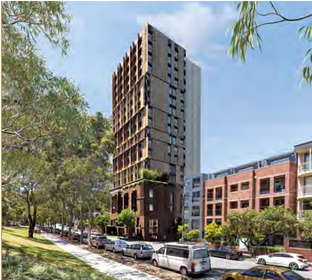
Property Name: Y Suites on Gibbons Location: 13-23 Gibbons Street, Redfern Number of Beds: 472 Status: To complete in March 2023 and for operations in first semester of 2023
