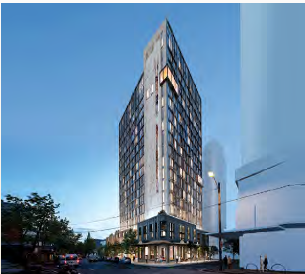
Property Name: Y Suites on Regent Location: 90-102 Regent Street, Redfern Number of Beds: 408 Status: To complete in November 2023 and for operations in first semester of 2024
