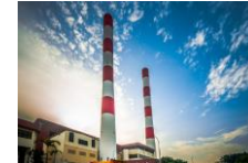
Senoko Waste-to-Energy (WTE) Plant
