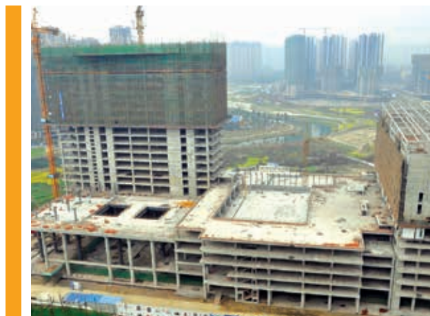
Ongoing construction of the Millennium Waterfront Chengdu Hotel
