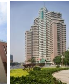
Somerset Olympic Tower Property Tianjin
