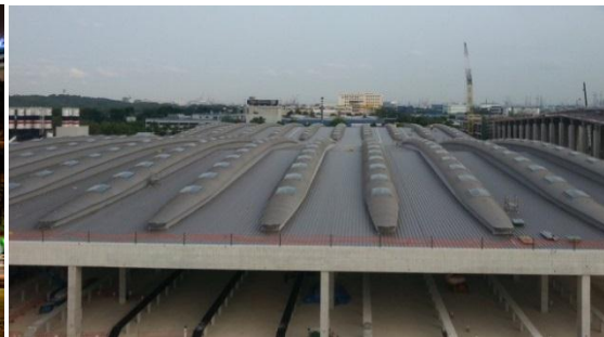
Tuas West MRT Extension Depot
