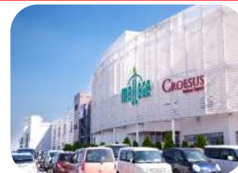
Mallage Shobu Suburban shopping centre in Kuki city, Saitama Pref.
