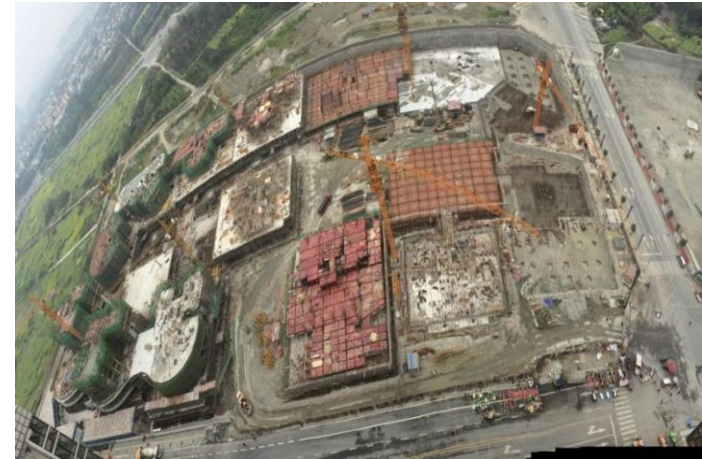
Aerial view of Plot A blocks under construction
