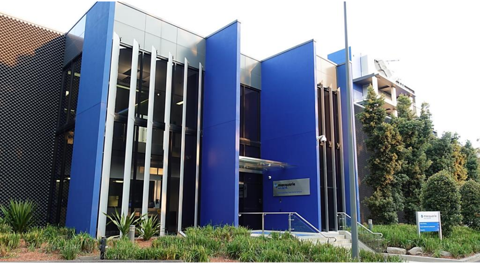
Intellicentre 3 East Data Centre
