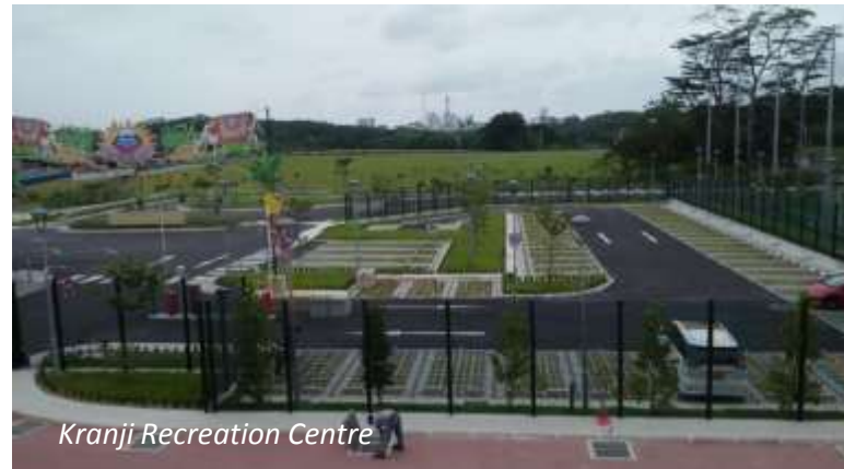
SolarNova 1 PV installation
