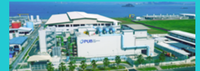
Tuas Desalination Plant.
