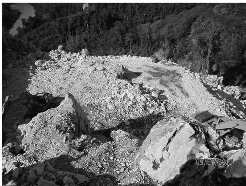
Figure 4-2; Excavation at Level 3 of Hill 2A
