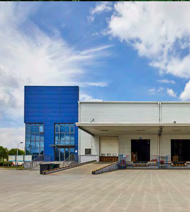
Initiated the installation of solar panels on the roof of Kunshan Bacheng Logistics Park
