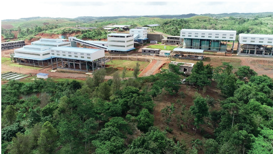
Figure 3. Wilton's 500 tonnes per day Flotation and Carbon-in-Leach mineral processing plant in Ciemas
