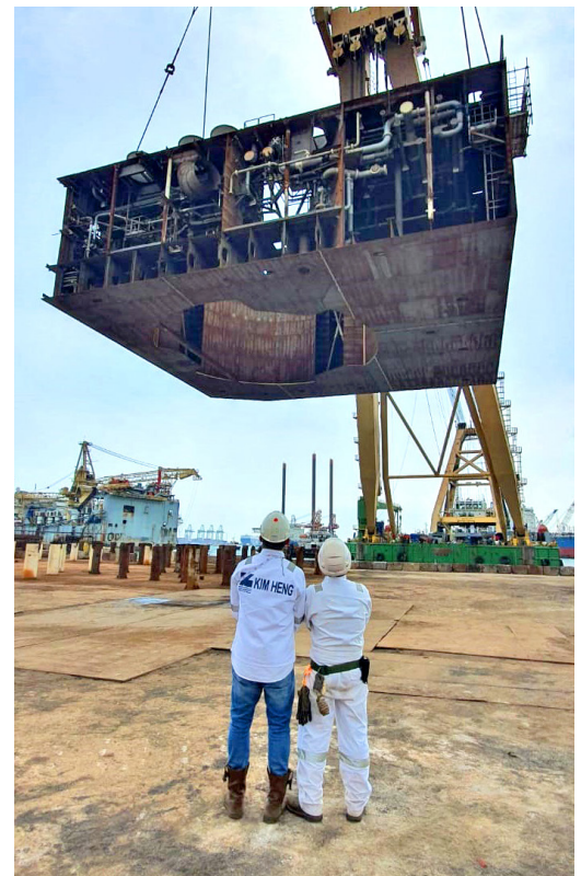
Heavy Lifting of Block
