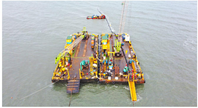
HDD Work Barges Working in Taiwan's offshore wind farm
