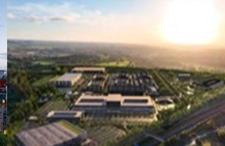
AiOnX data centre development fund
