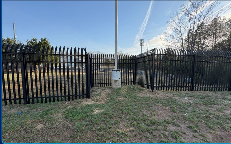
Installed New High-Security Perimeter Fence
