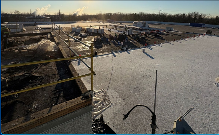
Replaced Existing Roof
