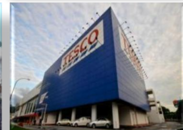
TESCO Building Penang
