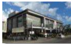
Siloam Hospitals Bali
