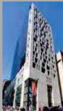
77 King Street Office Tower, Sydney
