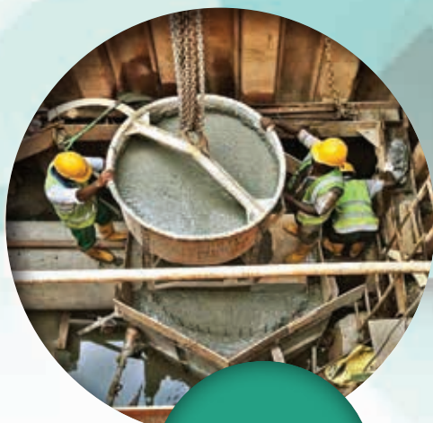
Casting of manhole chamber in one of our pipelines project.
