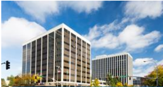
The Plaza Buildings, Seattle
