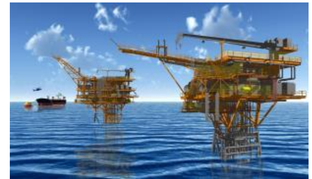
The Nong Yao oil development will comprise 20 development wells and two platforms producing to a nearby FSO
