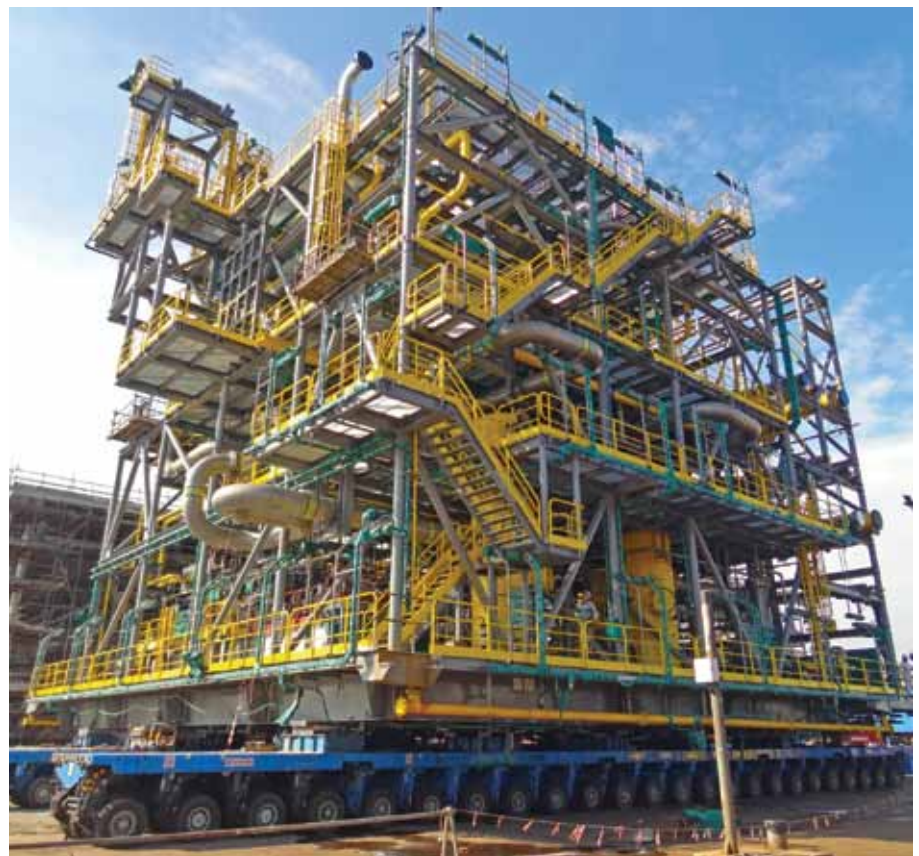
Successful completion and load out of Main Compression A module for FPSO Cidade De Saquarema
