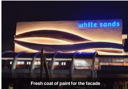
Fresh coat of paint for the facade
