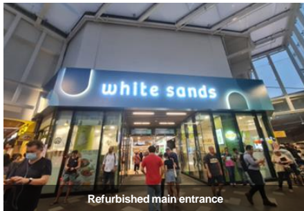
Refurbished main entrance
