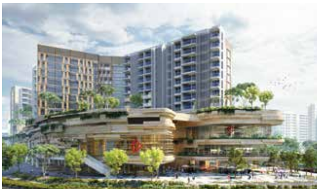
Sengkang Central, a mixed-use residential and commercial site in Singapore
