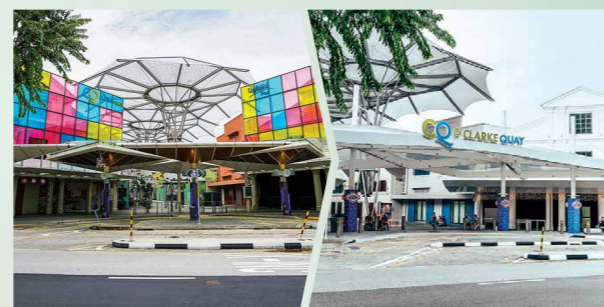
▲ Refreshed drop-off point and taxi stand at CQ @ Clarke Quay
