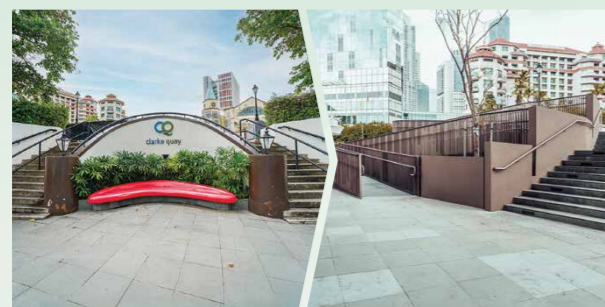
▲ The upgraded Read Bridge landing with a new accessibility ramp
