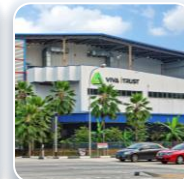
81 Tuas Bay Drive
