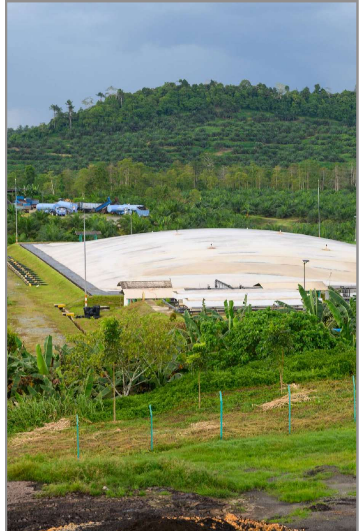
Methane capture plant in Sabahmas Mill, Malaysia
