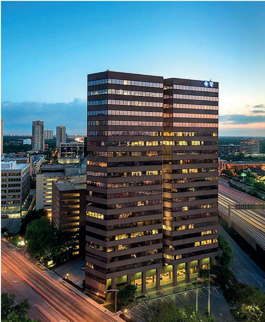
The Manager seeks to do its part for the environment through minimising the environmental impact and carbon footprint of the properties in its portfolio, which includes 1800 West Loop South (pictured).
