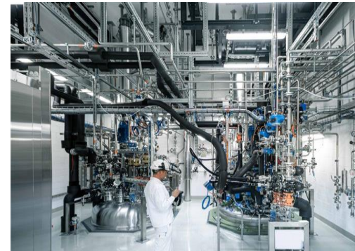
Existing Facility, Visp
