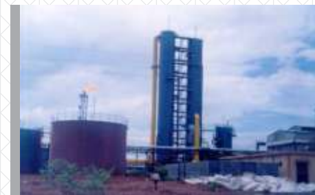
Ammonium Sulphate Plant – Konark Metcoke
