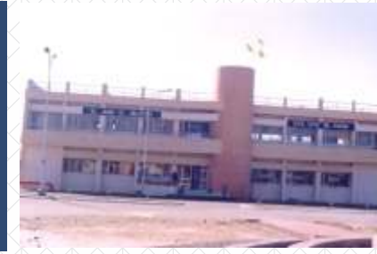
Civil Work – IOCL, Sangrur
