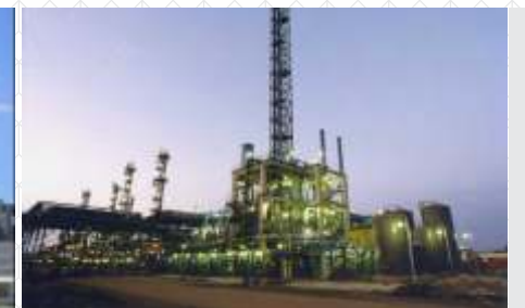
VCM Incineration Plant – IPCL, Gandhar
