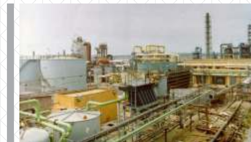
Desulphurisation Project HCL, Ghatsila
