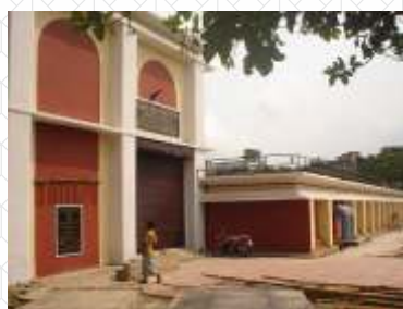
Booster Pumping Station at Kalighat Park – IRCON, Kolkata
