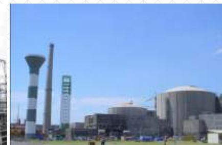
Heavy Water Upgrading Plant – NPCIL, Tarapore
