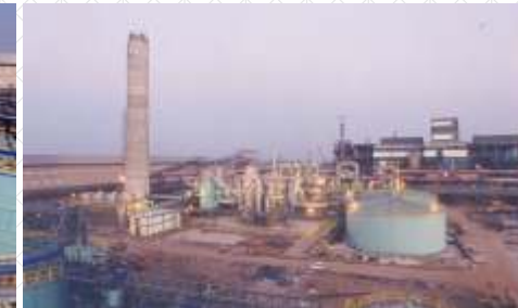
Sulphuric Acid Plant – Birla Copper, Dahej
