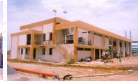
Civil Work for VVSPL Project – GAIL, Pata
