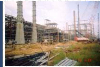
Hydro Cracker Project Chennai Petroleum, Chennai
