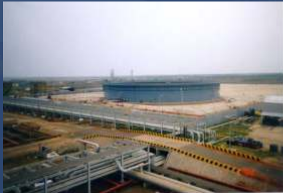
DDFR Tank – Cairn Energy, Rava Onshore
