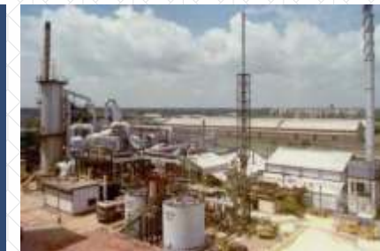
Sulphuric Acid Plant – HLL, Haldia
