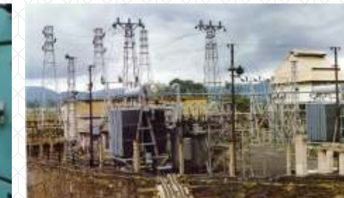
Electrical Work – NHPC, Jeypore
