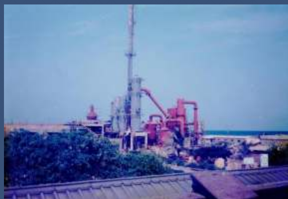
Sulphuric Acid Plant – EID Parry, Ennore
