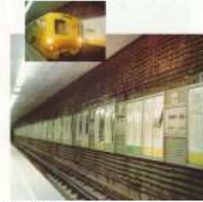
Cable Laying – Metro Railway, Kolkata
