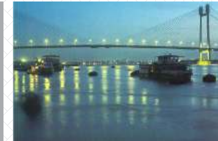
Illumination Work – HRBC, Kolkata
