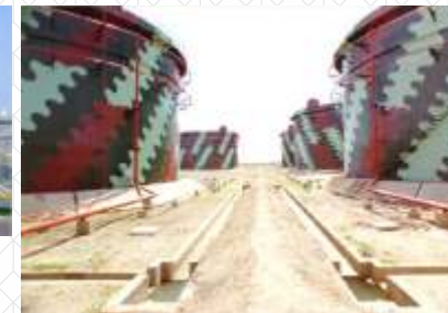
Tankage Work – ONGC, Hazira
