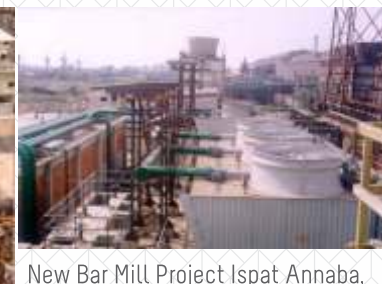
New Bar Mill Project Ispat Annaba, Algeria
