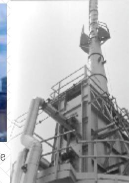
Naphthalene Purification Plant, SAIL, Durgapur
