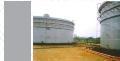
Tankage Work – Chennai Petroleum, Chennai
