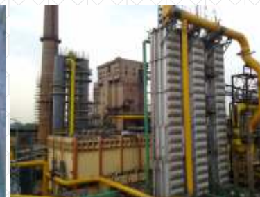
Gas Condensation Plant, SAIL – Burnpur
