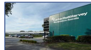
24 41-45 Hydrive Close, Dandenong South
