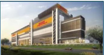
10 DHL Supply Chain ARC 1 Greenwich Drive
