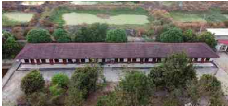
External View of the Subject Property (C1)
