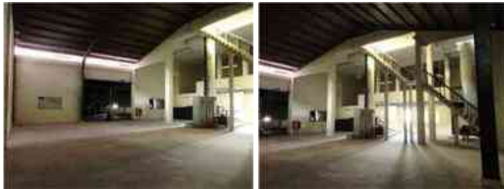
General View of the Ground Floor
