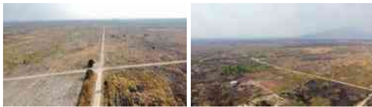
Other General View of The Subject Property
