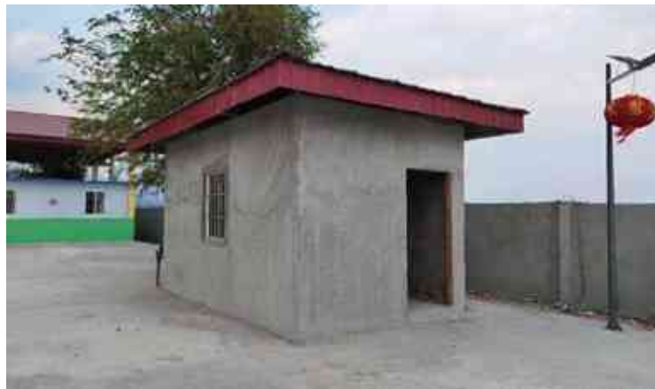
External View of the Security Guard (C4)
