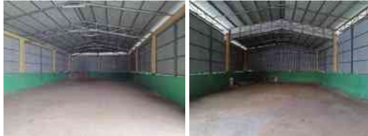
General View of the Subject Property (A1)
