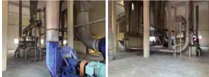
General View of the First Floor
