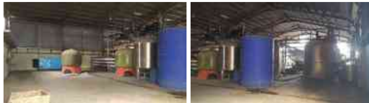
General View of the Subject Property (A1)
