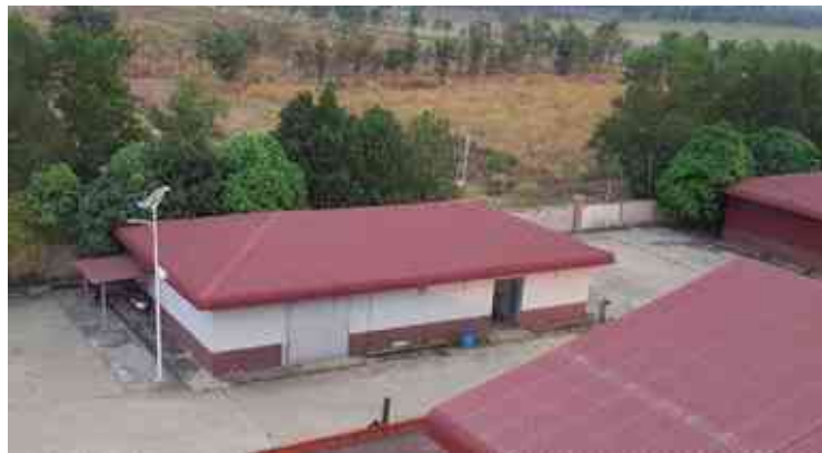
External View of the Subject Property (C2)
