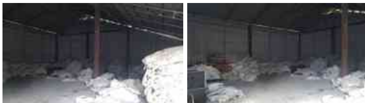
General View of the Subject Property (A4)
