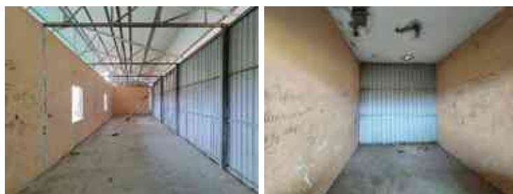
Other General View of the Subject Property
