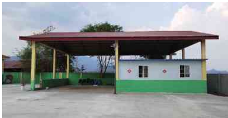
External View of the Covered shed (C5)
