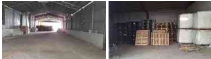
General View of the Subject Property (A2)
