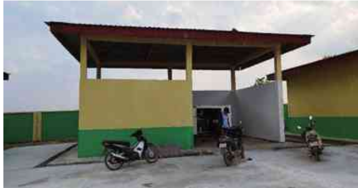
External View of the Generator Room (E3)
