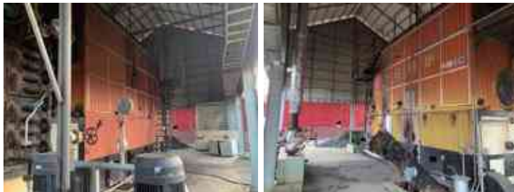
Other General View of the Subject Property (A3)
