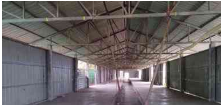
Internal View of the Storage (C1)
