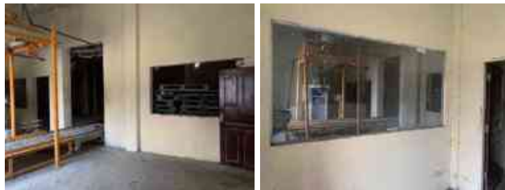
Other General View of the Ground Floor
