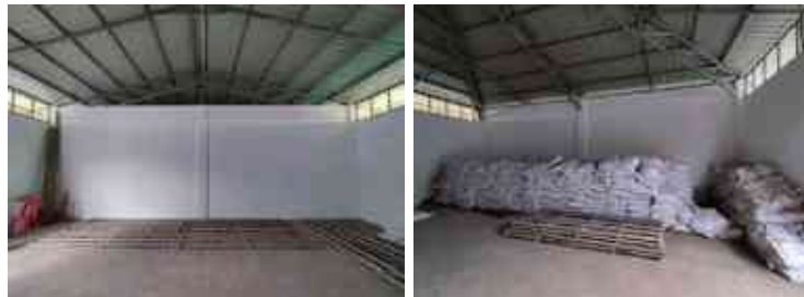
General View of the Subject Property (A2)
