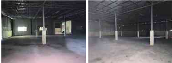
General View of the Subject Property (A3)
