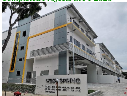
Tuas Bay Drive
