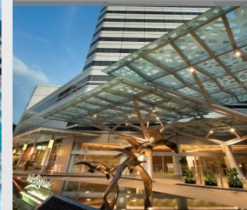
Raffles City Tower: Achieved AEI ROI of 9.3% p.a. in 2014
