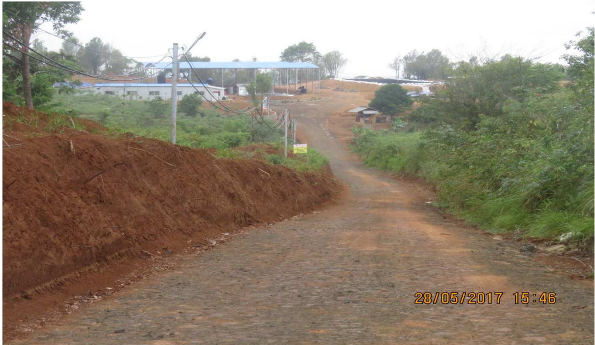
Hauling road and power supply to processing plant.
