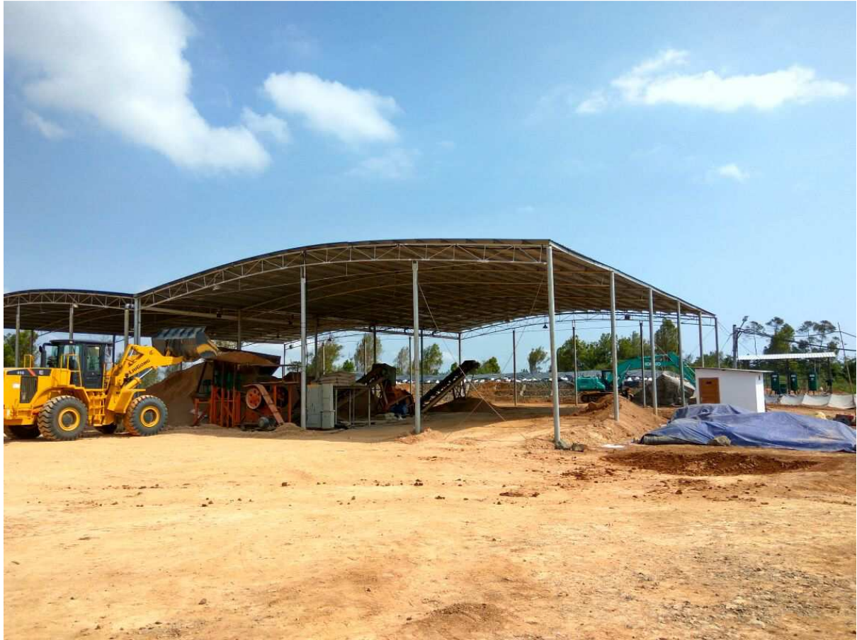
Processing area showing crushers and carbon absorption circuit at the background.
