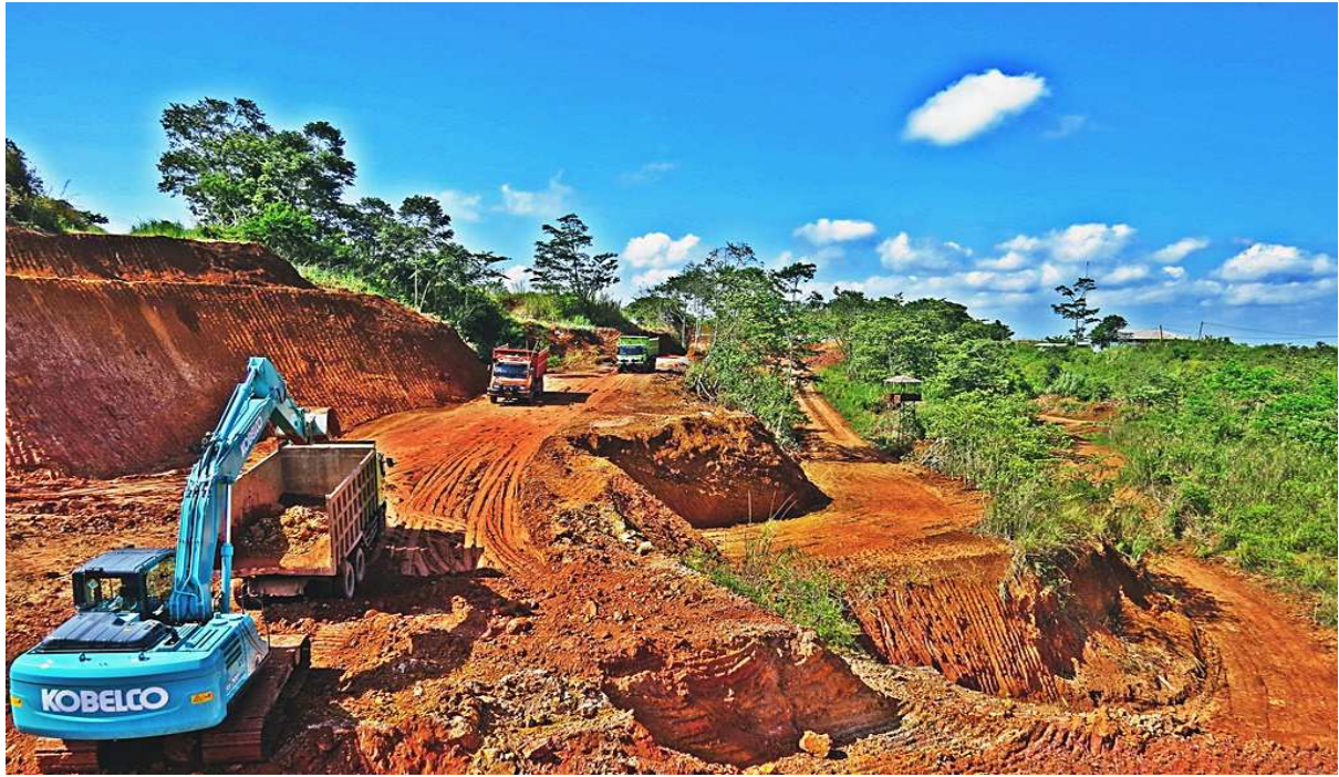
Stripping and mining.
