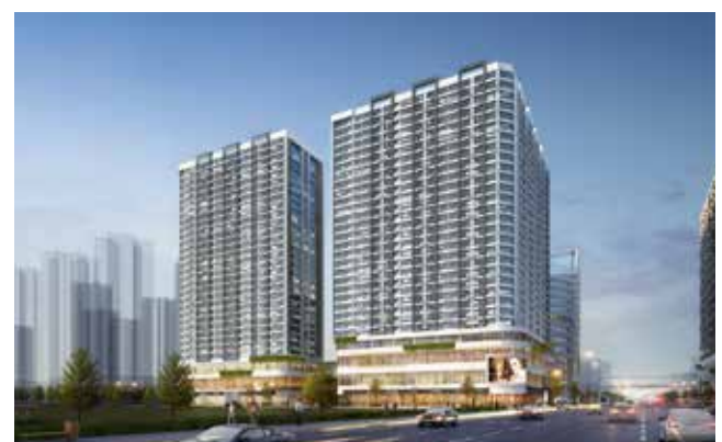
Millennium Waterfront Project, Chengdu, PRC
