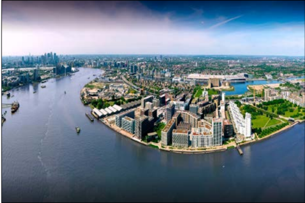
TOWNSHIP DEVELOPMENT Royal Wharf
